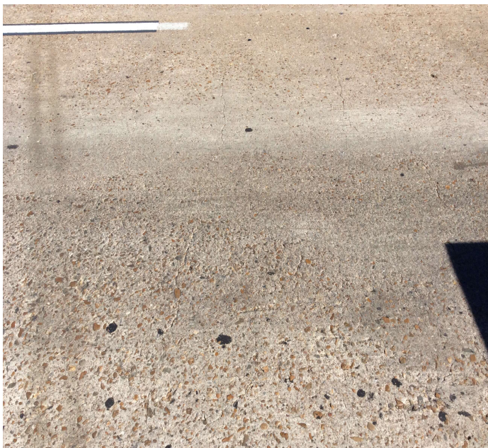
PHOTO 3 Description Typ. Cracking in Deck.
