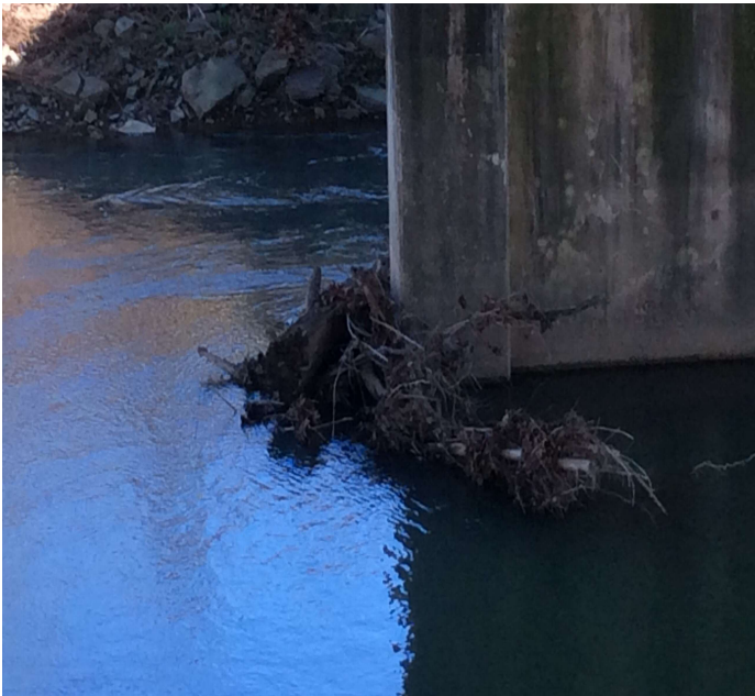
PHOTO 1 Description Drift at Pier 3.
