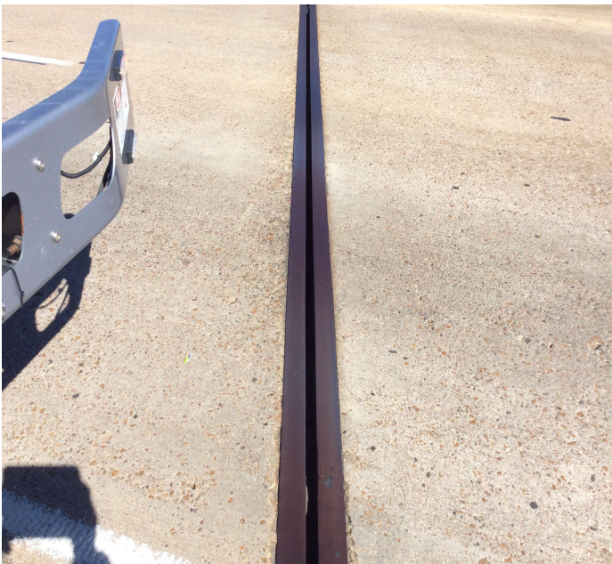
PHOTO 1 Description Seals Failed at Joints.
