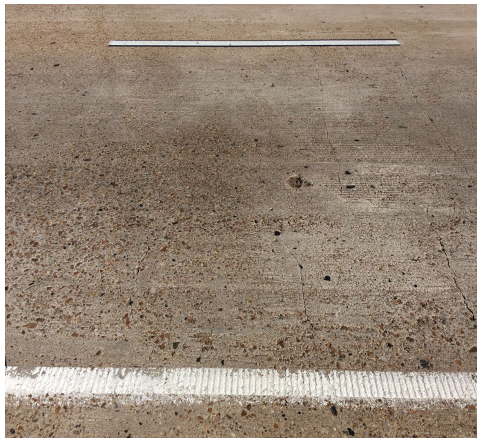
PHOTO 1 Description Typ. Cracking in Deck.
