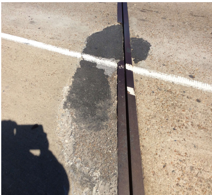
PHOTO 4 Description Patched & Spalled Areas at Joints.
