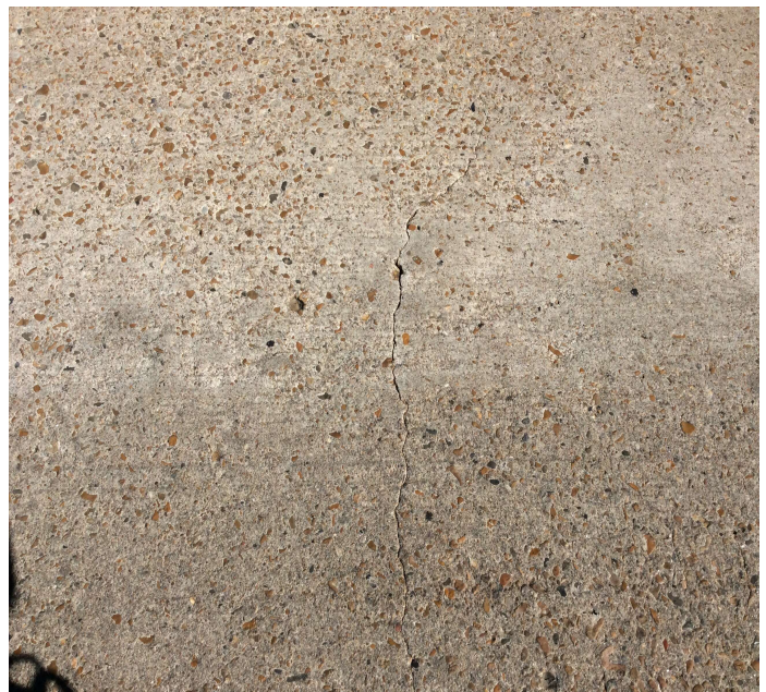
PHOTO 2 Description Typ. Cracking in Deck.
